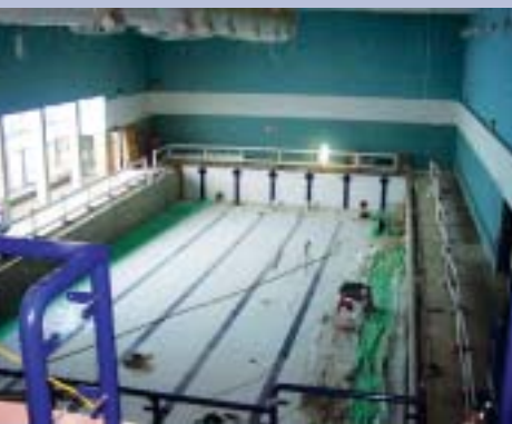
Construction of the 25m pool
